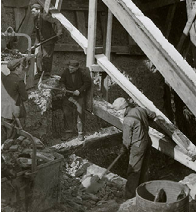
Construction of a masonry wall in Johnstown, Pennsylvania. Many of the jobs created in 1933–1934 were construction jobs for unskilled workers. (Records of the Work Projects Administration, RG 69)
